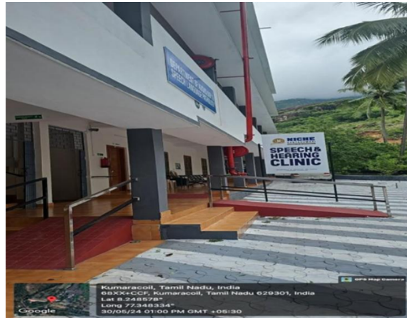
Fig. 9.12.1 Classrooms with ramps
